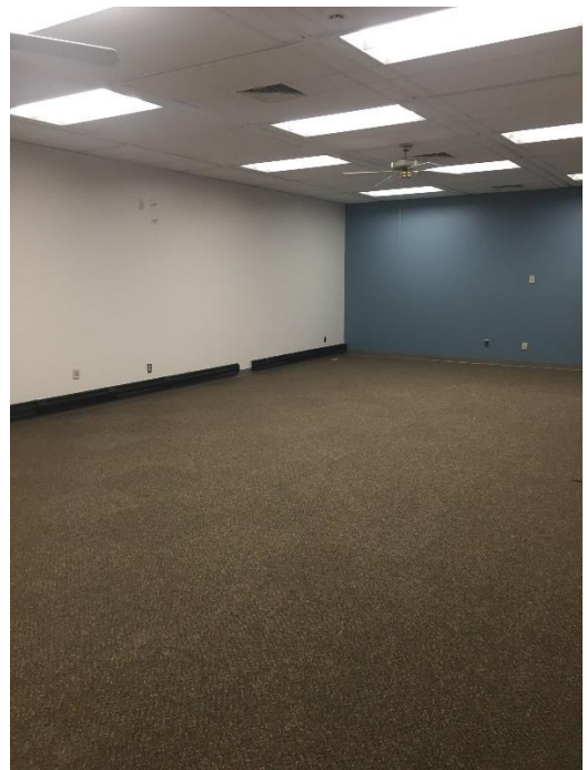
Board room after carpet and paint
