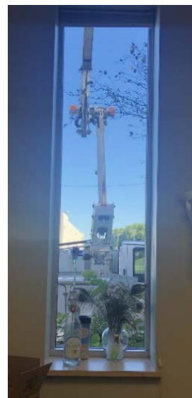
Security cameras being installed
